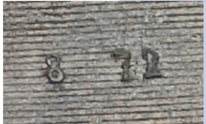
Belgian motorway E40/A3, built as a 20 cm thick continuously reinforced concrete pavement: in service for 50 years
