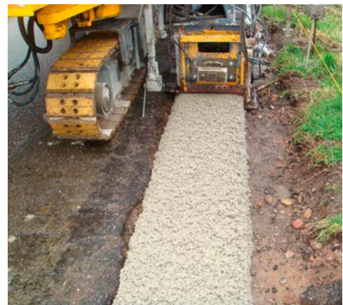
Construction of 'Bermcrete' in the Netherlands © Heijmans
