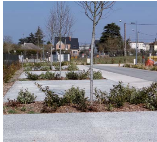
Car park with a pervious concrete pavement, Dreux (France) © CIMbéton
