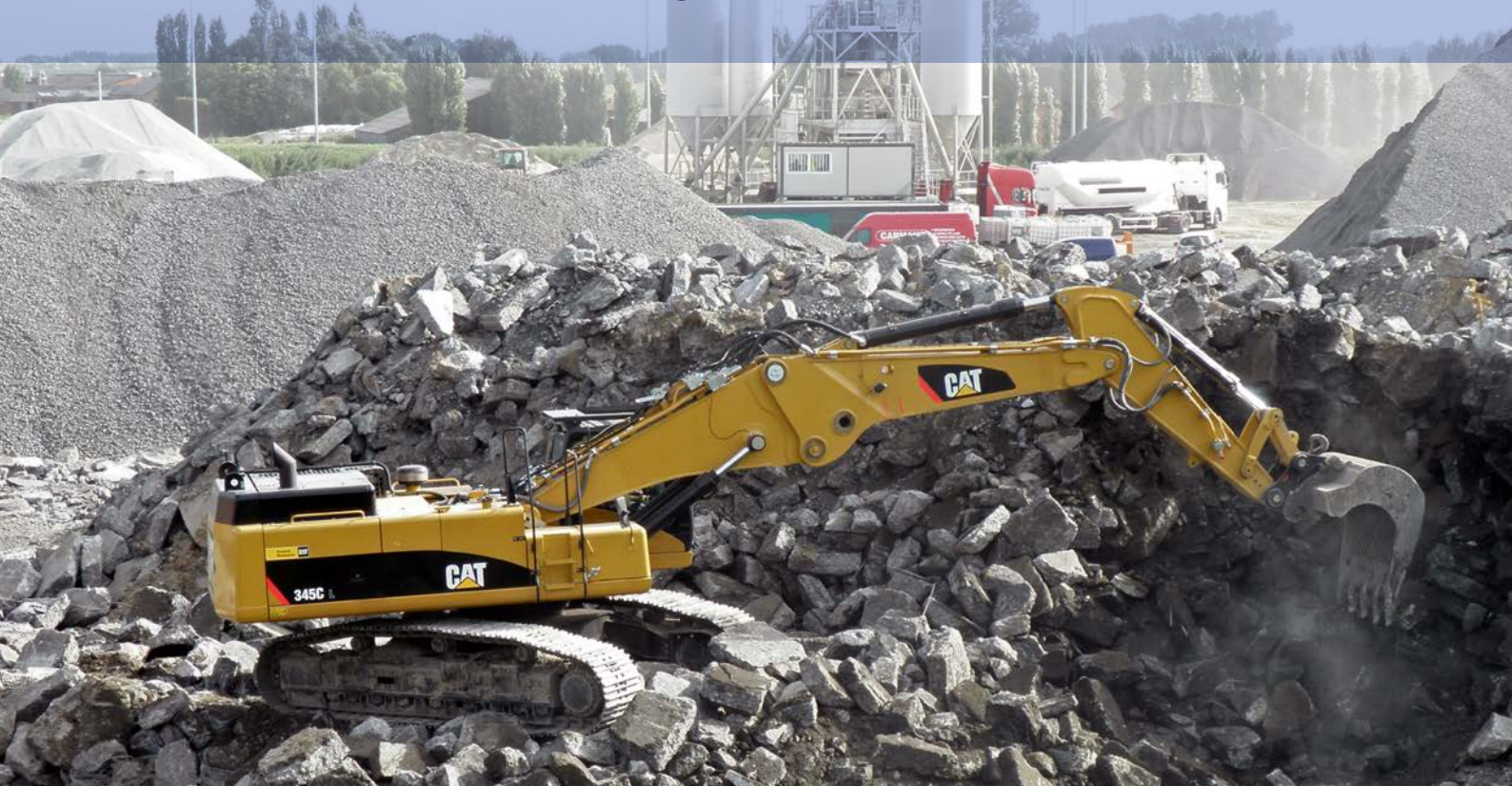
Concrete pavement recycling – motorway E17, De Pinte, Belgium, 2011 © L. Rens / FEBELCEM
