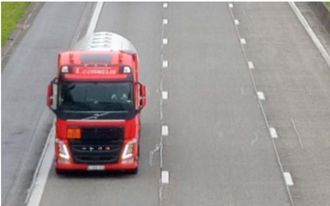
Belgian motorway E40/A3, built as a 20 cm thick continuously reinforced concrete pavement: in service for 50 years
