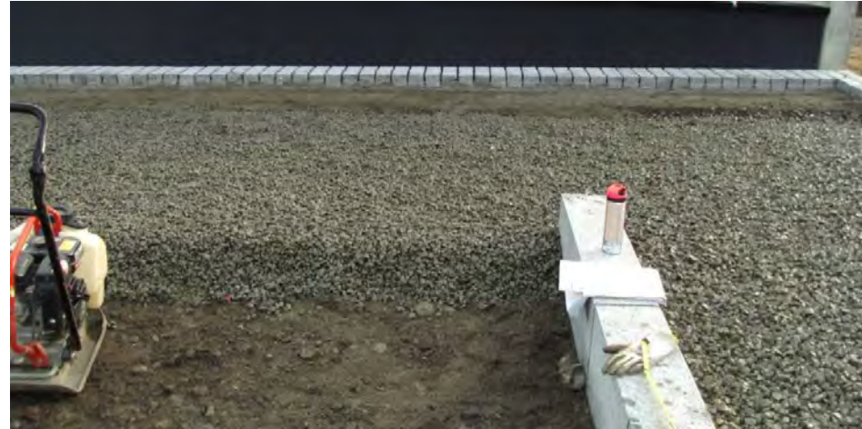
Sub-base for paving blocks
