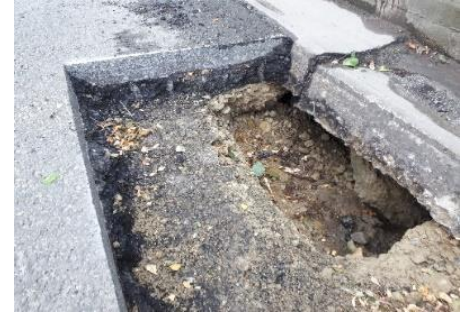
Large cavity under a kerb channel
