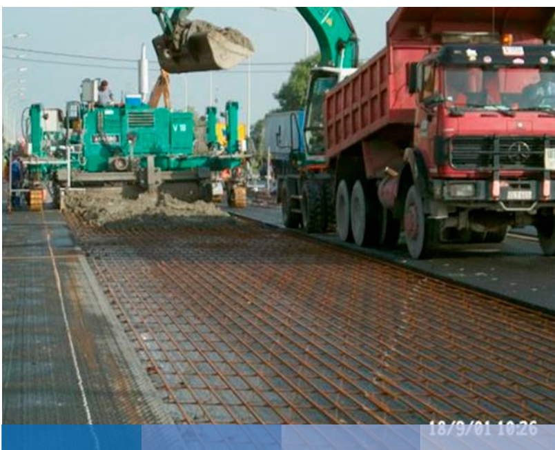
Figure 39. Construction of CRC inlay of asphalt pavement in Belgium (Rens, 2006).
