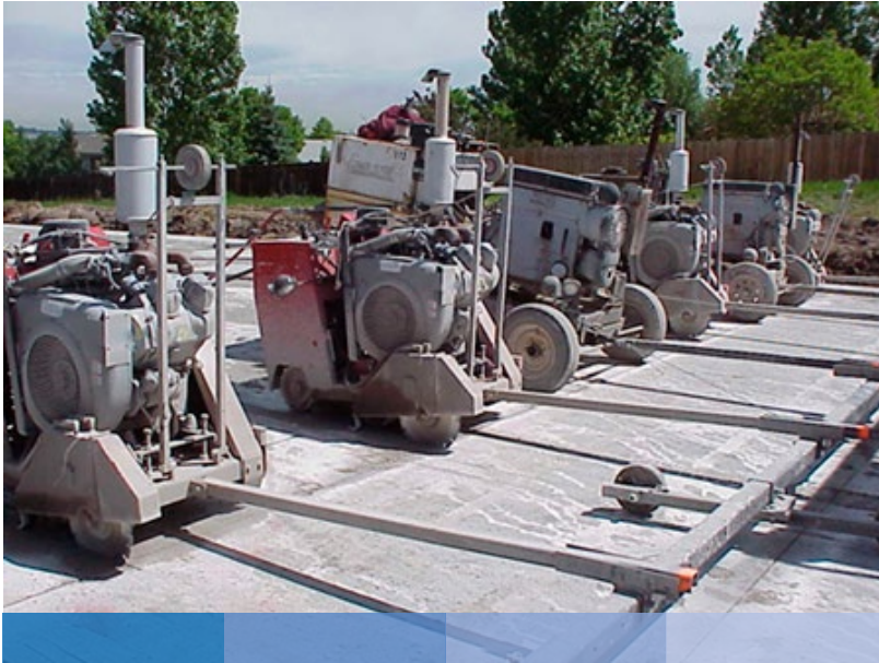
Figure 35. Many saws for sawing many joints. Snyder, 2019.
