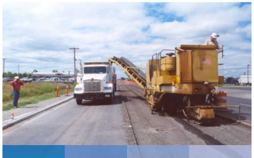
Figure 34: Milling of asphalt for profile and bond. Photos: Cimbeton 2004 (up) and U.S. National Concrete Pavement Technology Center (down)).
