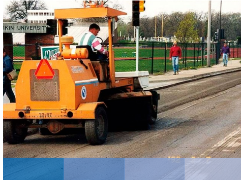
Figure 40. Cleaning milled surface with power broom (left) and water blasting (right). Images: U.S. National Concrete Pavement Technology Center, Iowa State University.
