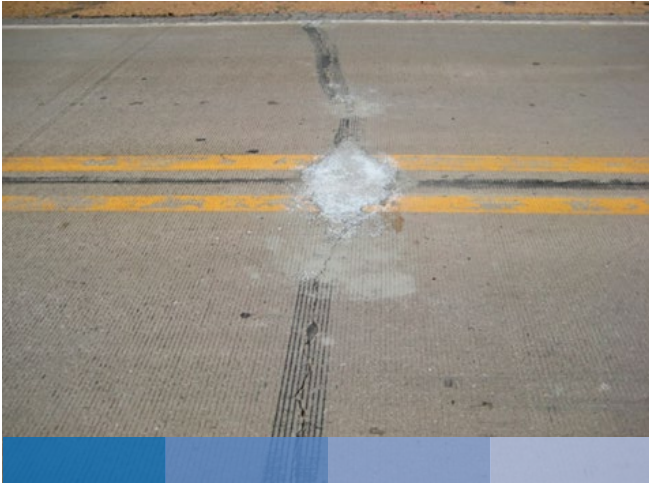
Figure 23. Examples pre-overlay repair of joint and crack spalling using cement-based mortar. Photos from Todd LaTorella, MO/KS Chapter of ACPA
