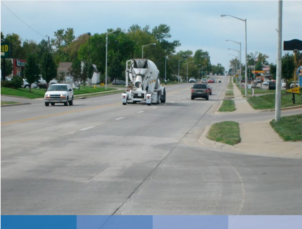
Figure 10. Example completed concrete overlay of concrete – bonded on US 56 in Kansas (USA). Photo: Todd LaTorella, MO-KS Chapter of ACPA
