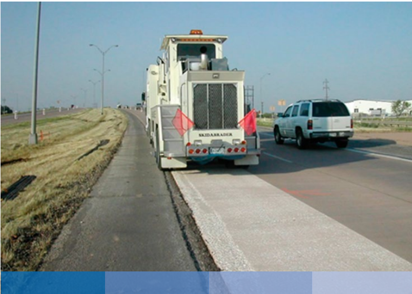
Figure 17. Milling concrete for bonded concrete inlay (Spalt 2015).
