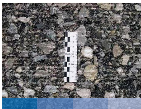
Figure 41. Image of cleaned, milled asphalt surface (Riffel 2010).
