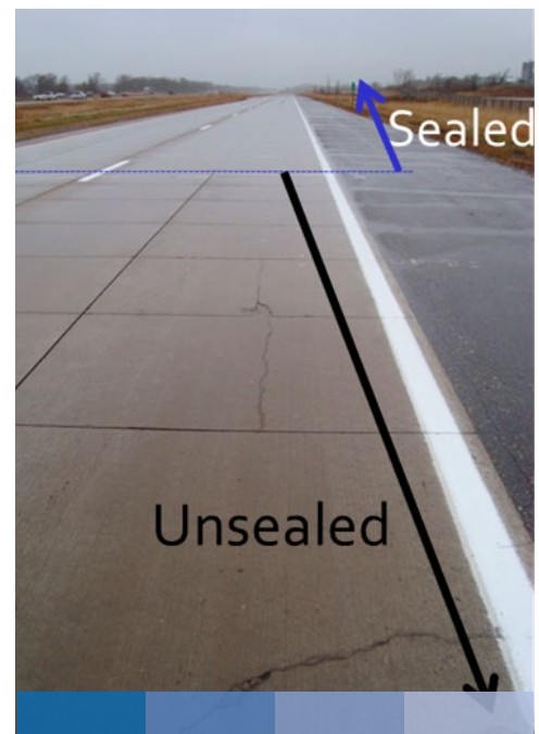
Figure 37. Differences in COA-B performance in Minnesota (USA) for sealed and unsealed joints. Photo: Tom Burnham, Minnesota DOT.
